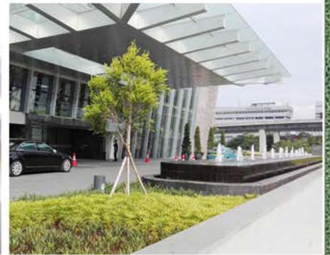
GAMA TOWER, JAKARTA
